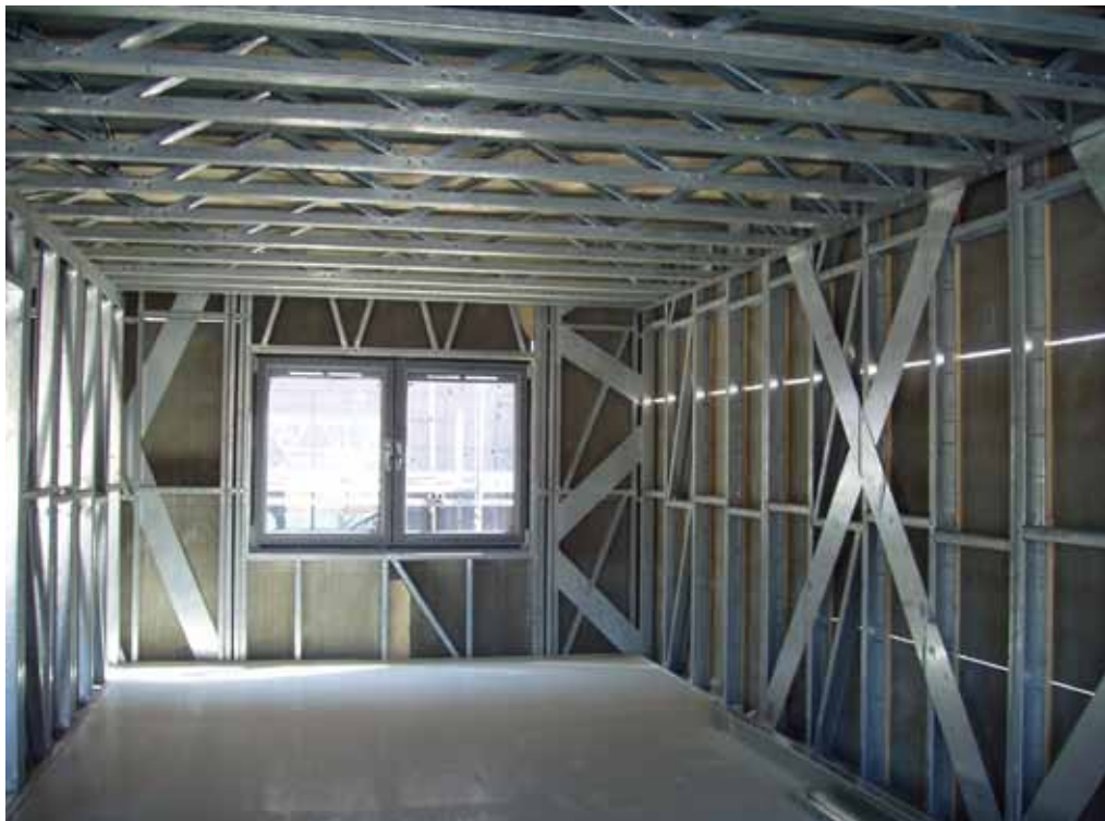
Figure 5 Light steel frame showing floor cassette and wall frames
