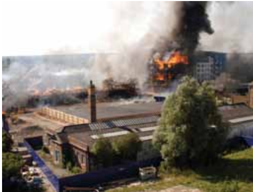
Figure 32 B3 (east elevation) collapse and fire spread to B2 (reproduced by courtesy of the London Fire Brigade)
